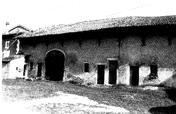
Lorraine farm built of earth brick in four bays, with roof overhang supported on brackets. Vallée de la Meuse.
