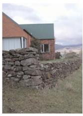
The new wall was built in 1996 from freshly gathered up field stones. It is 65 metres long and is a full-depth dry stone wall with an 800 mm thick base. The bottom stones are sitting on clay. The new house behind has 52 piers going into this clay to counter the seasonal heave - clay swells when wet and shrinks when dry. The extent of this shows up as wide cracks in the surface of the ground.
