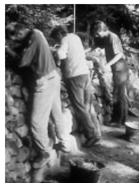
Rebuilding the drystone walls of the Cévennes terraces
