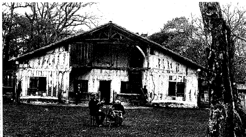
Gable facade of an early 19th century métairie with central recessed porch. Landes, Gascony.
