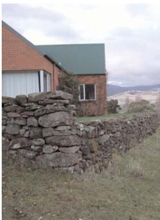
The new wall was built in 1996 from freshly gathered up field stones. It is 65 metres long and is a full-depth dry stone wall with an 800 mm thick base. The bottom stones are sitting on clay. The new house behind has 52 piers going into this clay to counter the seasonal heave – clay swells when wet and shrinks when dry. The extent of this shows up as wide cracks in the surface of the ground.
