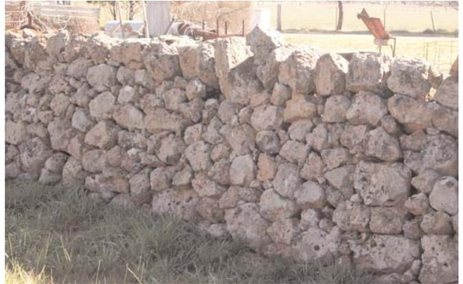
*Round heavy basalt stone was used to build this wall on the Rigbetti farm at Yandoit*
