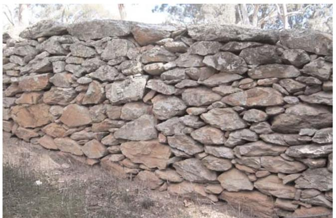
*Sandstone from the reefs was used to build this wall on the Gervasoni farm at Yandoit*
